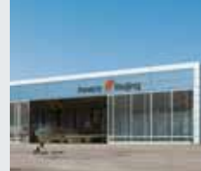
Ameco A380 Hangar Peking, China
